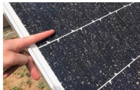
Figure 2: Cleared arid soils are difficult to stabilise, restore and revegetate (top); PV panels soiled from dust pollution (bottom).
